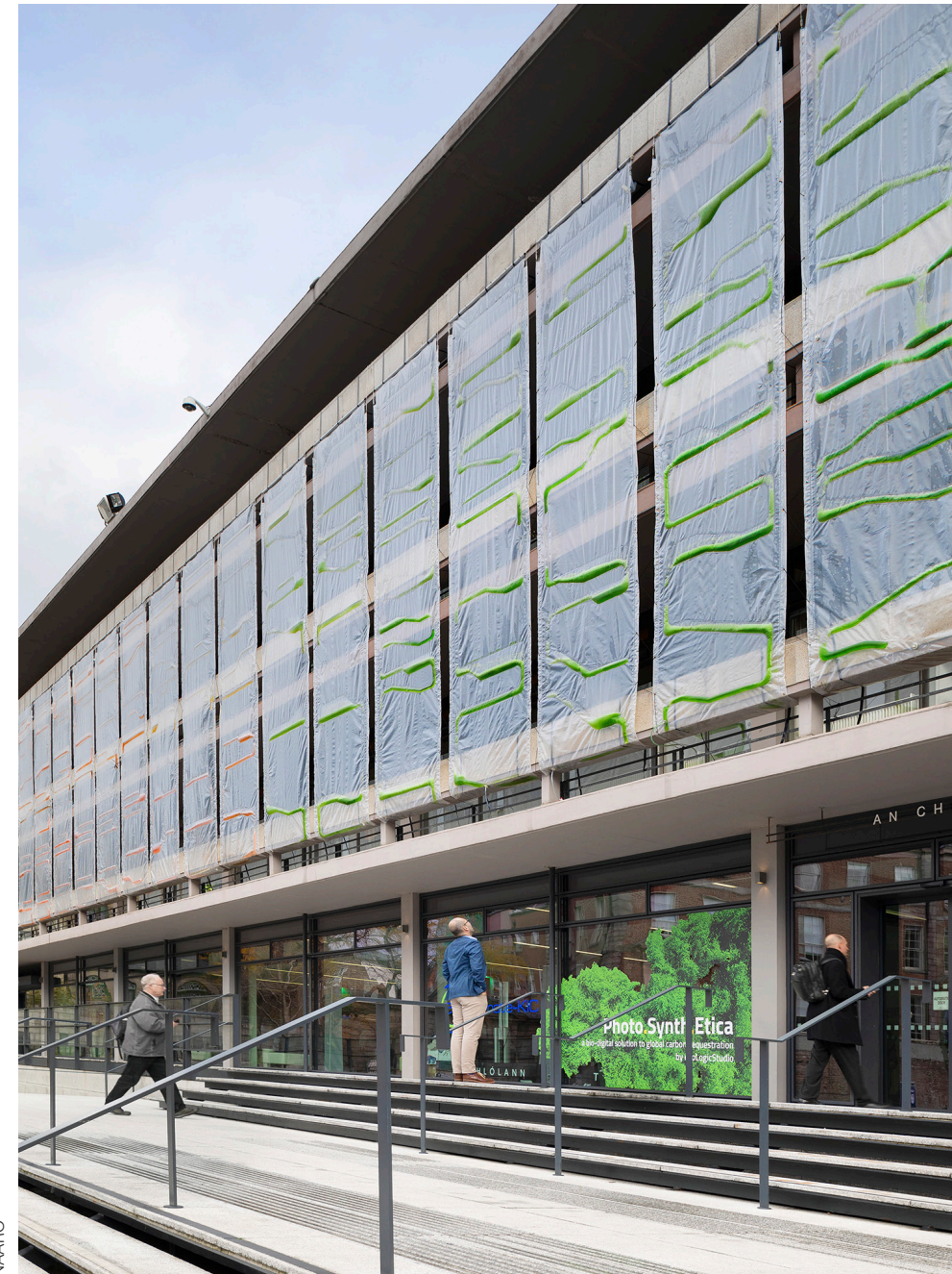
Designed for EcoLogicStudio's first collaboration with Climate-KIC, the EU's most prominent climate innovation initiative, and presented in Dublin during the week of the Climate Innovation Summit 2018, Photo.Synth.Etica is an 'urban curtain' that captures CO 2 from the atmosphere and stores it in real time.
